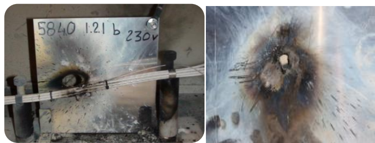
Figure 2.3-2 - Short circuit damage to structure: 230 V no tripping (left) vs 3000 V tripping in tens of milliseconds (right)
